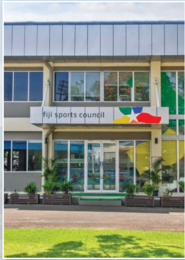
COVER The transformed headquarters for the Fiji Sports Council enhances service delivery to our customers and provides improved working conditions for staff.
